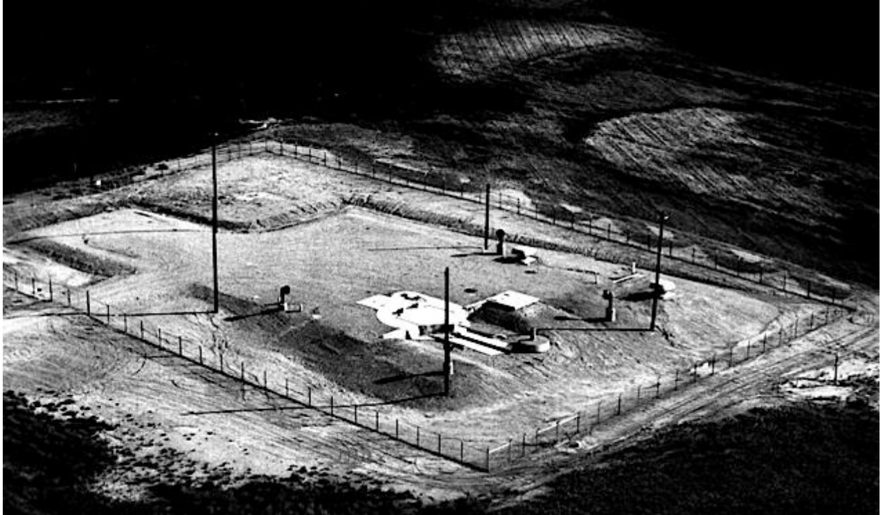
Typical unmanned Minuteman missile Launch Facility.
