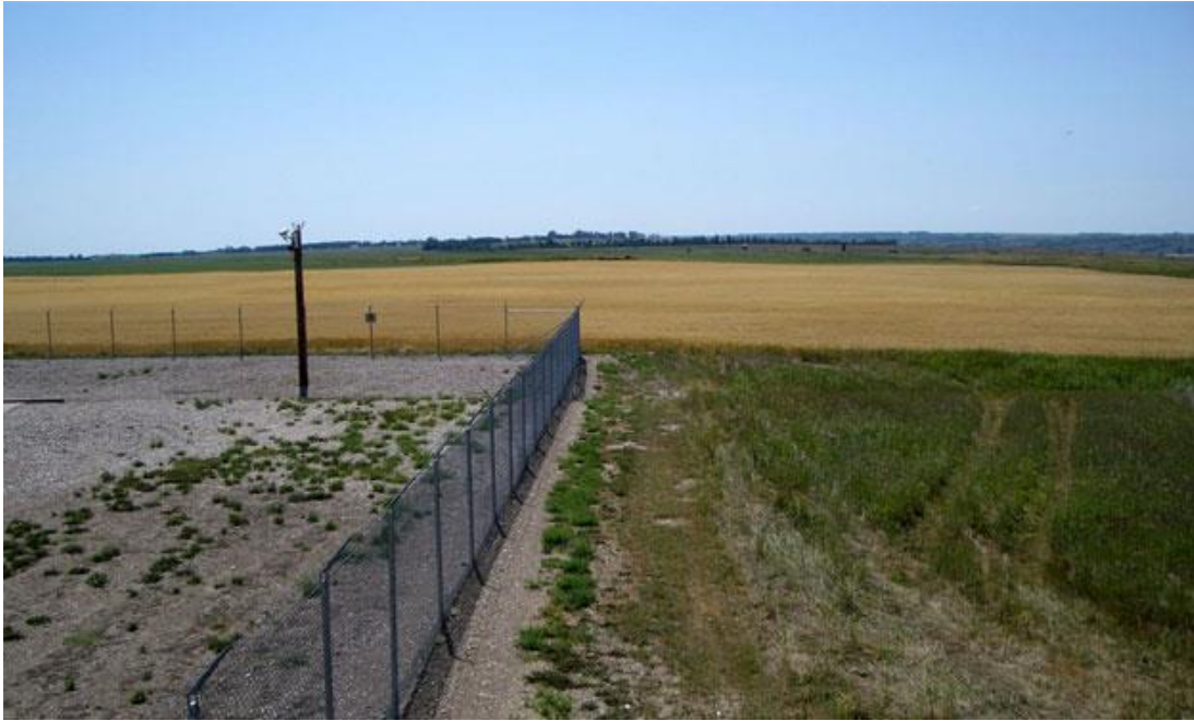
N-7 looking south from the front gate.
